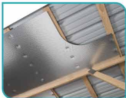
UNDER DECK INSULATION
